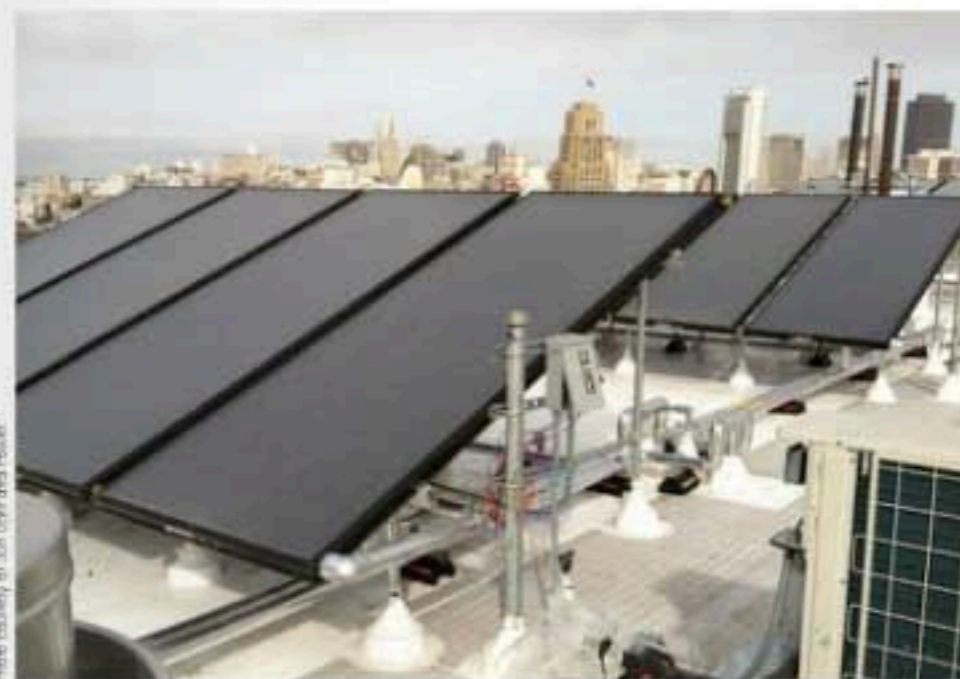
There are 38 solar panels on the roof at AVA 55 Ninth that help pre-heat the water flowing to the domestic hot water system. The solar hydrothermal system helps the complex meet California's Building Energy Efficiency Standards.
