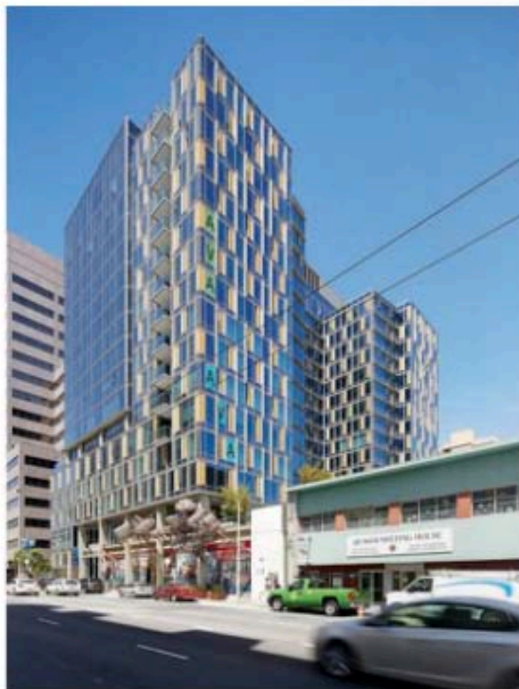
The AVA 55 Ninth complex is certified LEED Gold and features low-flow faucets, showerheads and toilets in all 273 units and common areas.
